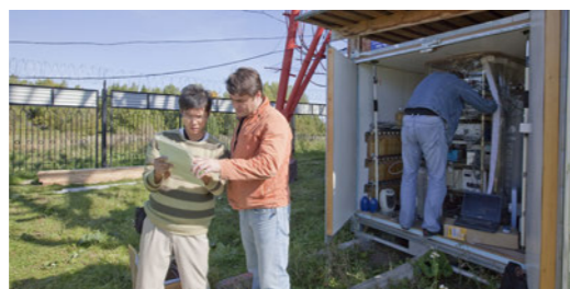
Maintenance of the tower observation system in Siberia
