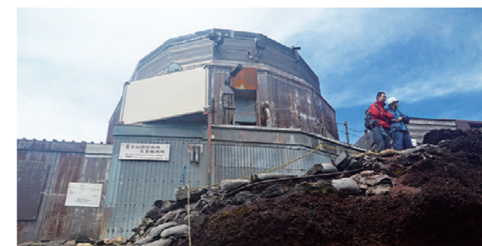
Special regional climate monitoring station on the top of Mt. Fuji
